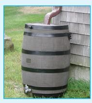
A rain barrel is a device which is available for home owners who have external downspouts and want to store rainwater to help water plants, wash a car, and help prevent stormwater runoff into the weeping tiles of their home. Rainwater can be diverted away from the foundation of the home and into the natural environment through the rain barrel extended release hose.
